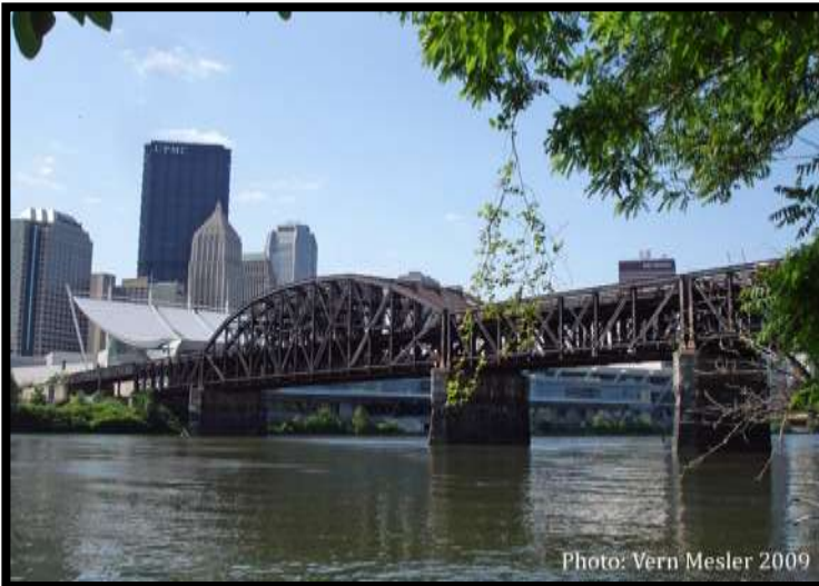
Fort Wayne Railroad Bridge
