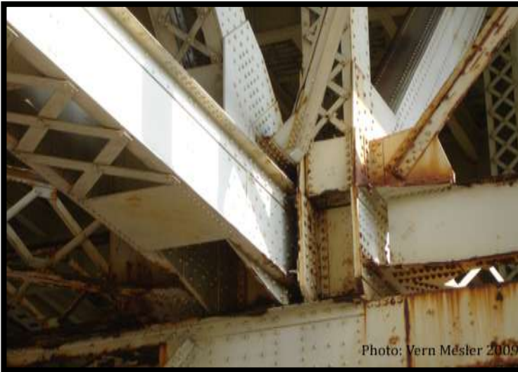
Liberty Bridge riveted connection
