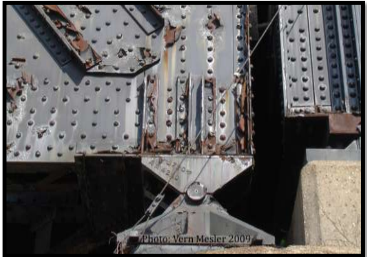
Panhandle Light Rail Bridge bearing pad
