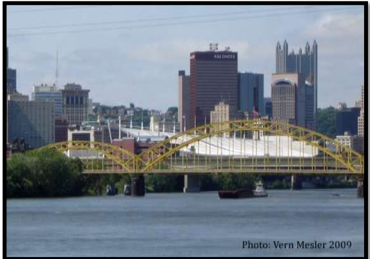
Sixteenth Street Bridge
