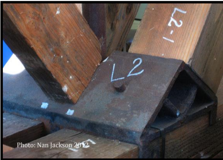
Timber diagonal fit to original cast iron shoe from the Moose Brook Bridge
