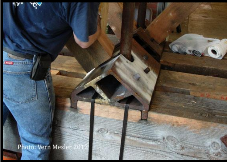
Timber diagonal positioned against a braze welded cast iron shoe
