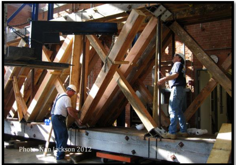
Crew members from Barns & Bridges of New England assembling the second Moose Brook Bridge timber truss
