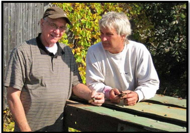
October 10, 2010 Vern Mesler and Nels Raynor inspect rivets and bolts used in the connection plates during the erection of the McIntyre Bridge.
