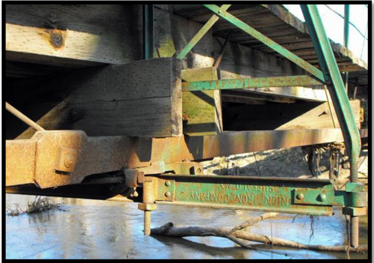
November 8, 2009 Vern Mesler and Nathan Holth photograph the unique wrought iron and cast iron structural members of the bridge. Notice the mill mark "Union Iron Company Buffalo NY"
