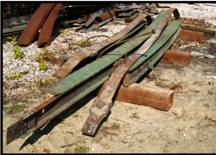
October 10, 2010 sections of the McIntyre Bridge in storage at BACH Ornamental & Structural Steel in Holt Michigan ready for the process of restoration. As a first step, a set of drawings will be produced for structural analysis.
