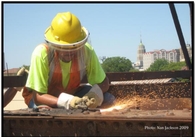
Guillermo Gonzalez removes rivet with a scarfing tip
