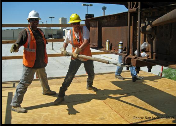
Jacob Loza and Guillermo Gonzalez remove a nut from an u-bolt
