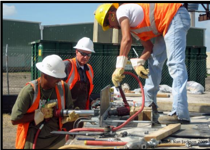
Driving rivets, Jacob Loza, Vern Mesler, and Guillermo Gonzalez
