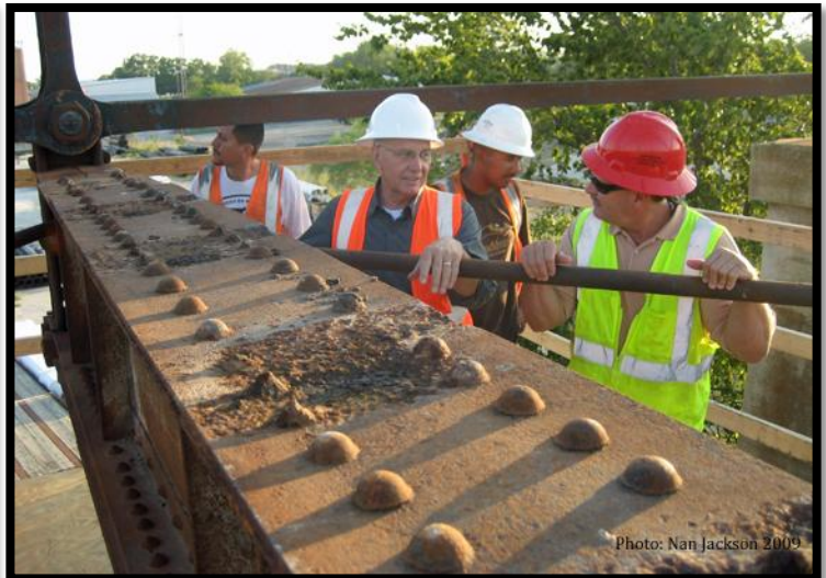
Riveted floor beam inspection
