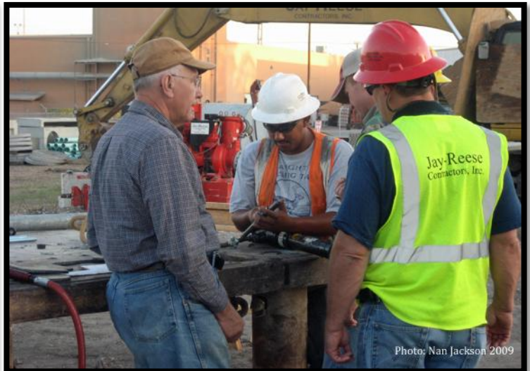
Setting up the rivet buster, Vern Mesler, Jacob Loza, Andrew Roberts, Lowell Burge
