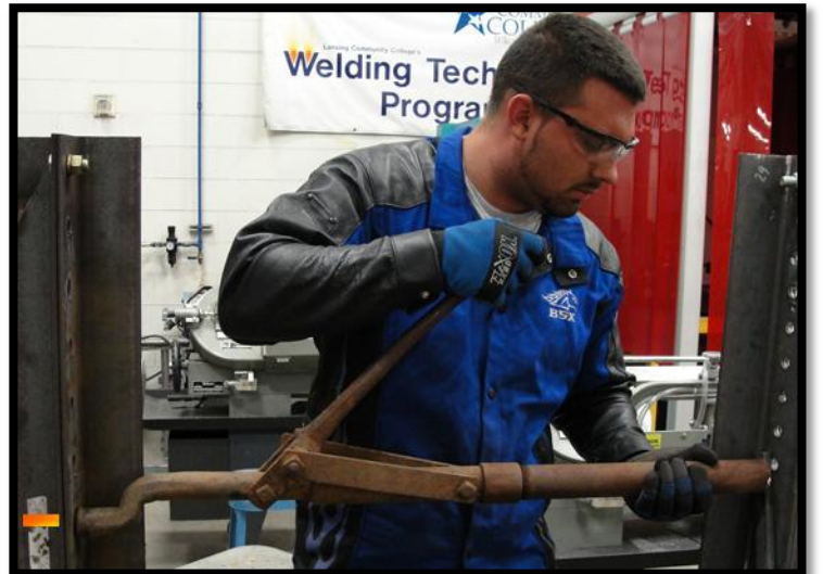
After positioning the working end of the holder-on over the manufactured head of the rivet, Mena secures the holder-on against the bracing.
