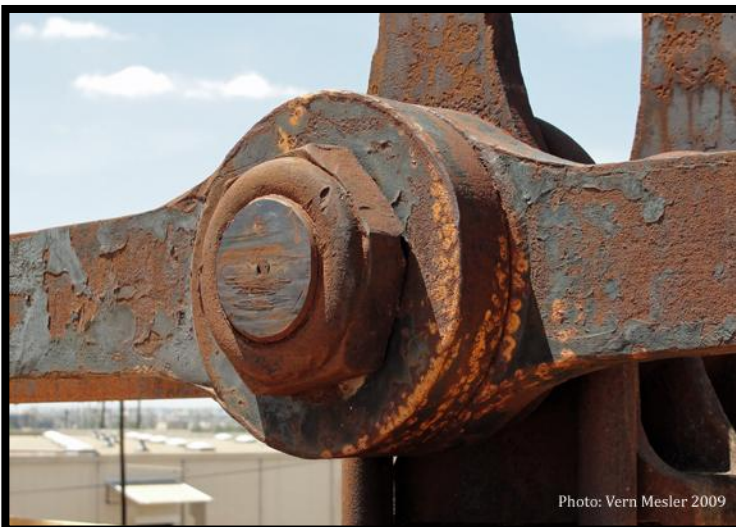
Phoenix-style eyebars are made from wrought iron
