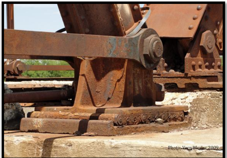
Original wrought iron rollers will be replaced
