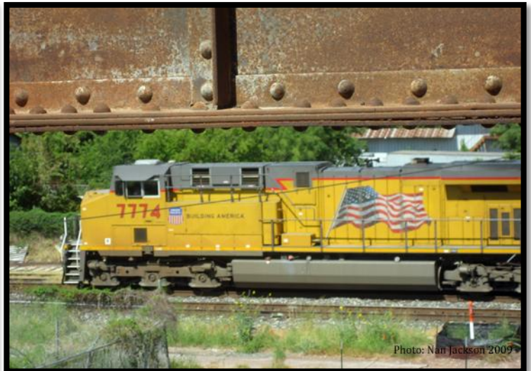
Hays Street Bridge crosses a still-active railroad
