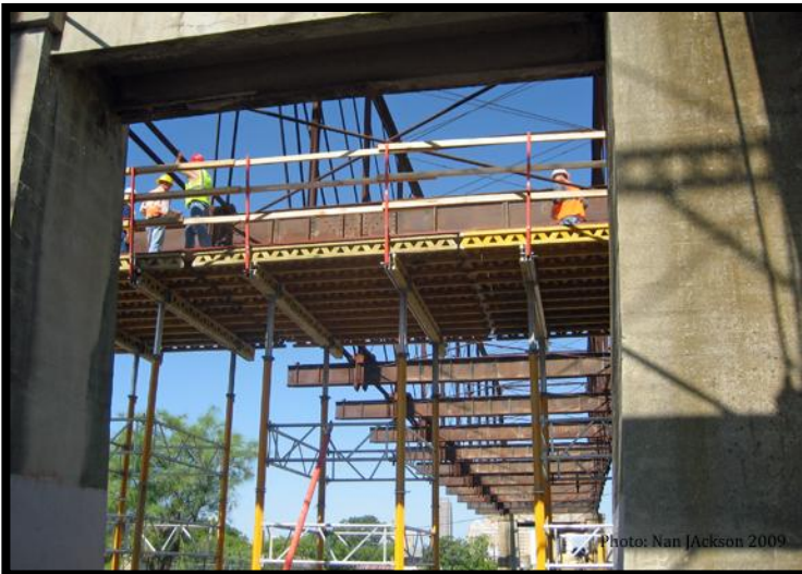
Engineer Patrick Sparks and others inspect a floor beam
