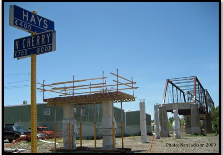
Approaches to the bridge will be concrete piers and span
