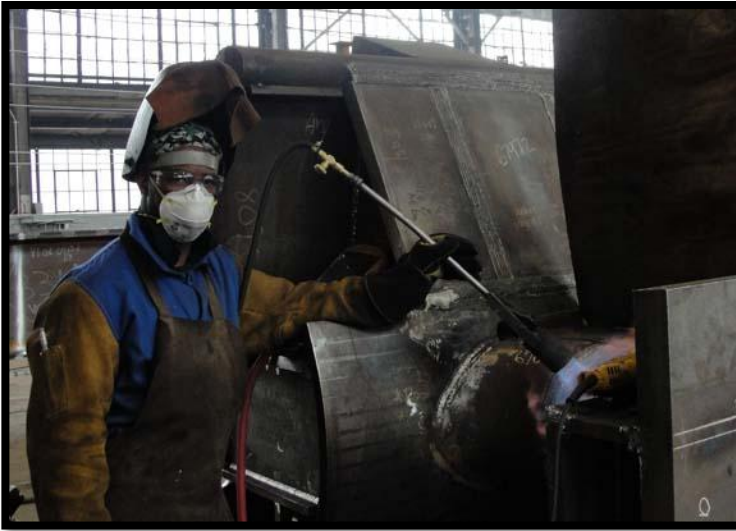
Welding operator preheats large section in preparation for welding
