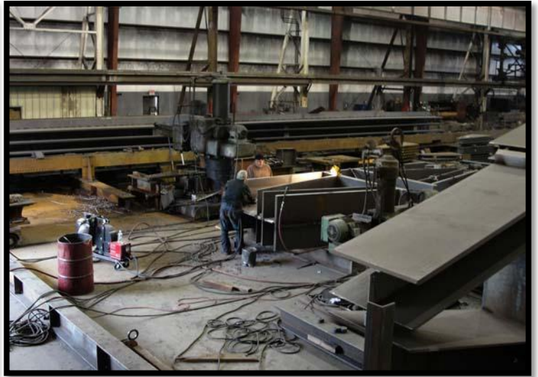
Fabrication of sections for World Trade Center site Transportation Hub
