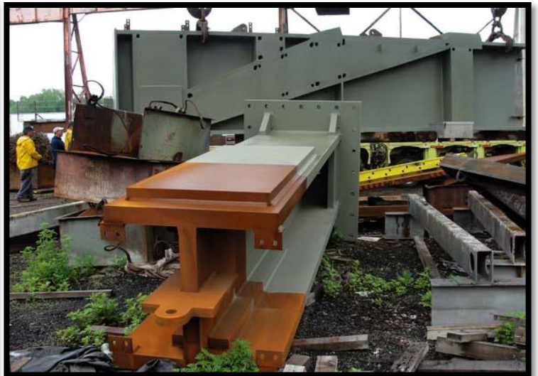
more fabricated sections for WTC at Harris Steel
