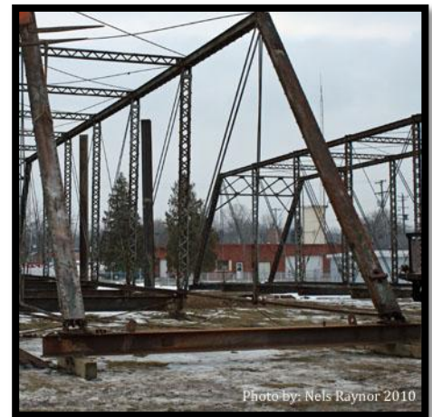
Dismantling began in January in preparation for primer painting and restoration
