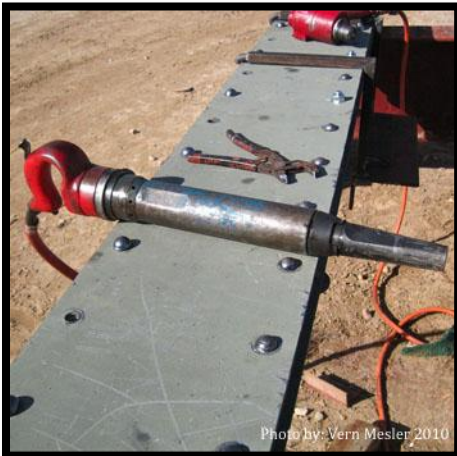
#60 Boyer field rivet hammer on a riveted top chord cover plate
