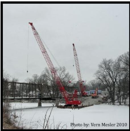
State Street Bridge prepared for removal from its original abutments
