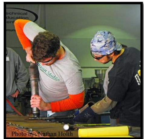
Dan Stinson assists a scholarship recipient with hammering out pack rust.
