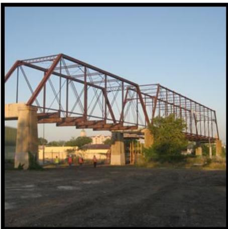
Hays Street Bridge with the 130ft Pratt Truss Bridge in the foreground and the Whipple truss in the background.
