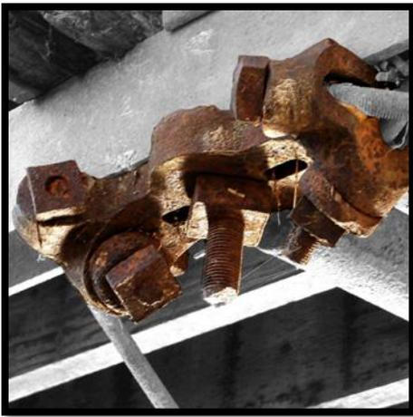
Cast iron connection member on the McDowell Bridge (*background has been changed to black and white in order to highlight the connection detail*)
