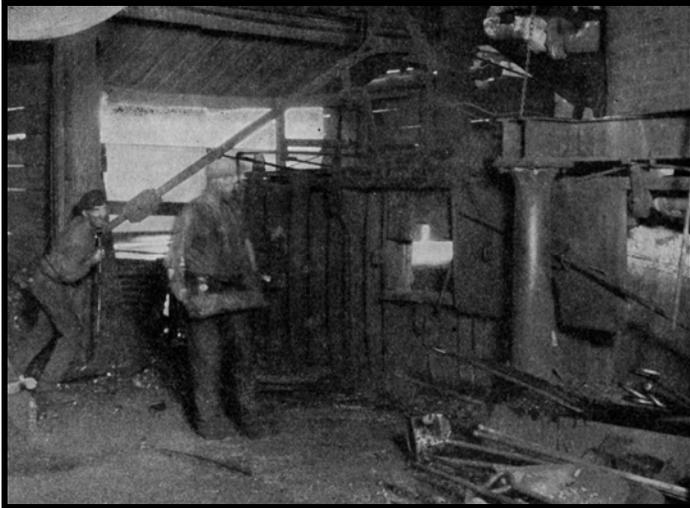
*Charging the puddling furnace with pig iron*
