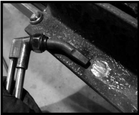
*Removing rivets with the oxygen fuel gouging tip for rivet restoration*
