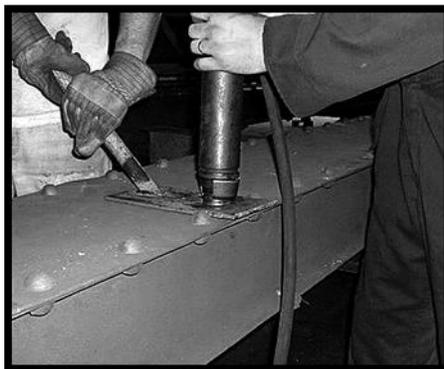
*Pack rust removal, heating and hammering*
