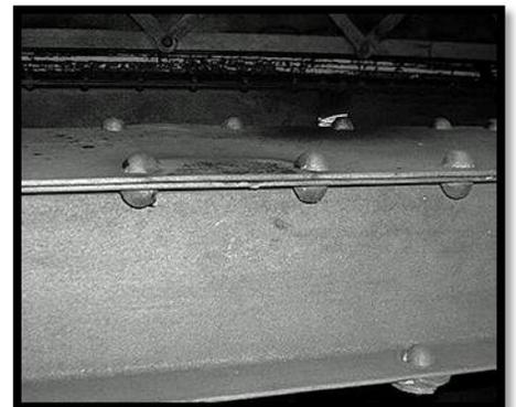
*Restoration of metal damaged by pack rust*
