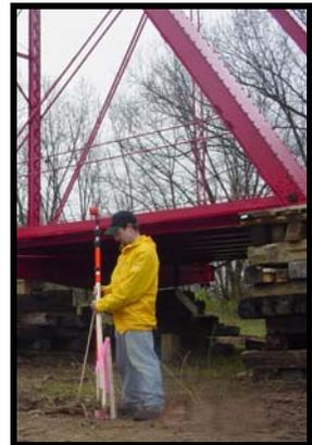
*Engineering Technician from Civil Engineers, Inc. lays out the East side abutment*
