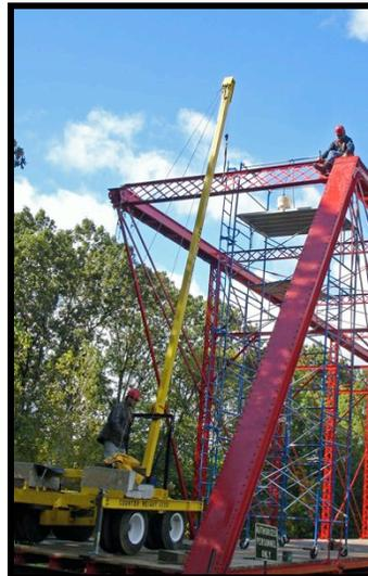
Conklin and Denniston lift in place with the gin pole the first inclined end post and portal. (Summer 2006)
