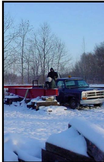
Conklin and Denniston lay out and punch holes in the floor beams to bolt the stringer beams in place. (Winter 2006)
