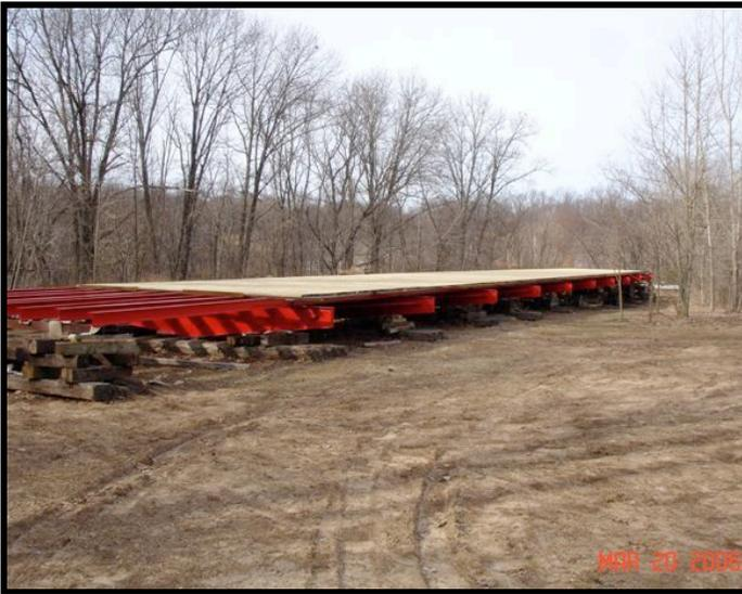
During the spring of this year Conklin and Denniston began installing the wood deck on the replicated floor beams of the Charlotte Highway Bridge in preparation for putting up the trusses. The gin pole was also being fabricated at this time with the help of Frank Hatfield, P.E. Professor Emeritus, Civil and Environmental Engineering, Michigan State University. On May 24<sup>th</sup> it was placed on the deck.
