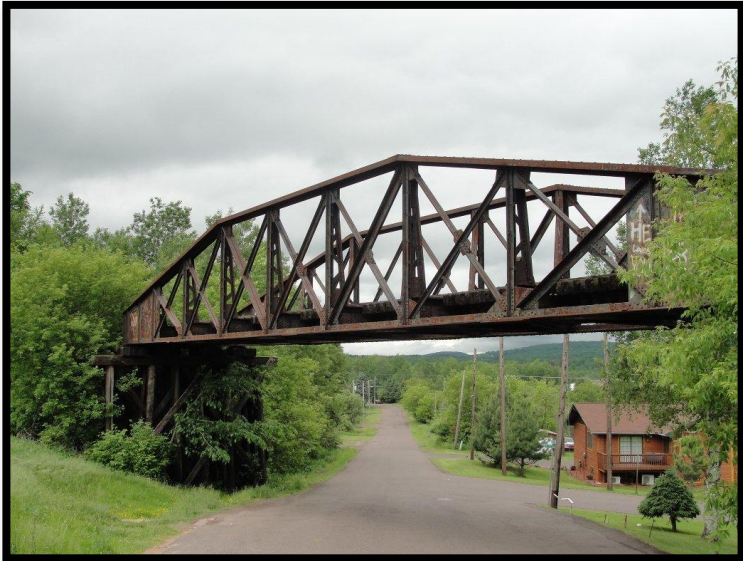
1st Ave railroad bridge, Bessemer
