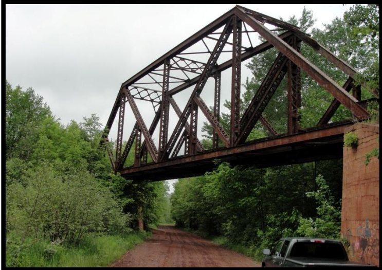
Soo Line railroad bridge over the old Chicago-Northwestern railroad bed
