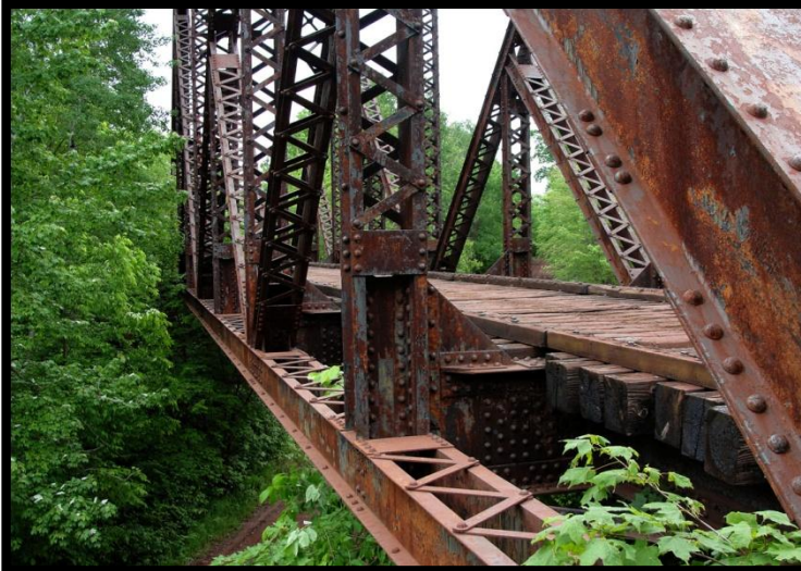
Soo Line railroad bridge
