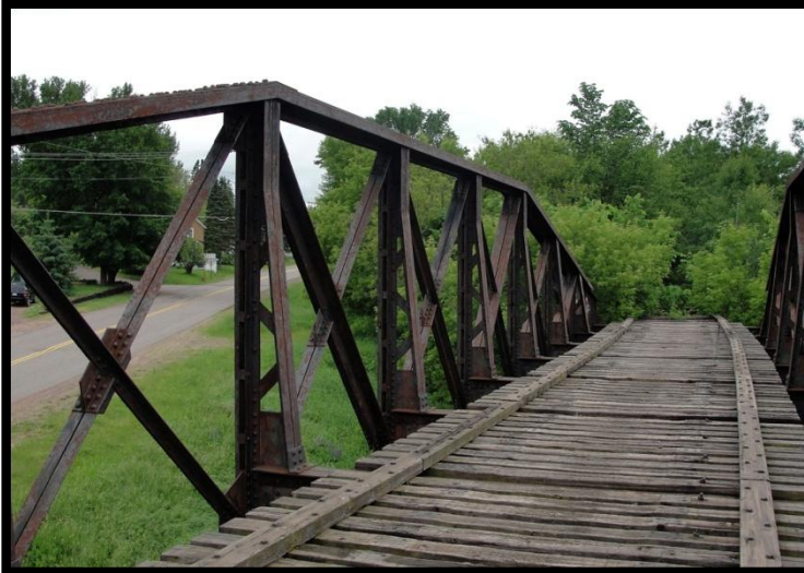
1st Ave railroad bridge, Bessemer
