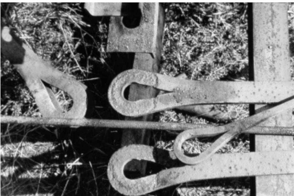
Figure 5. Forge-welded loop eyebars like these are obsolete.
