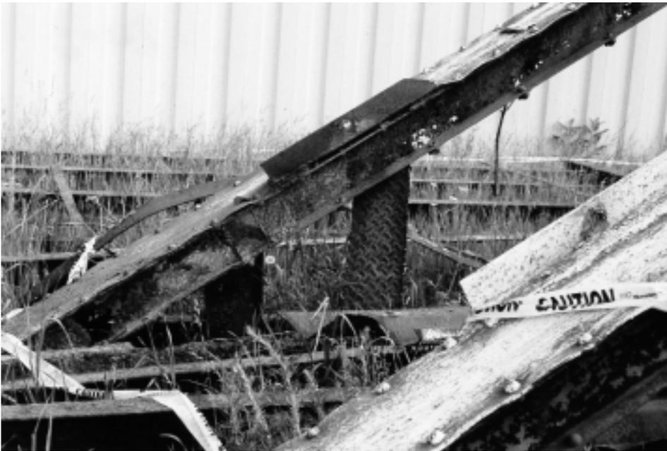
Figure 4. Severely corroded sections of the Twenty Mile Road bridge were replaced by welding new steel to sound original material.
