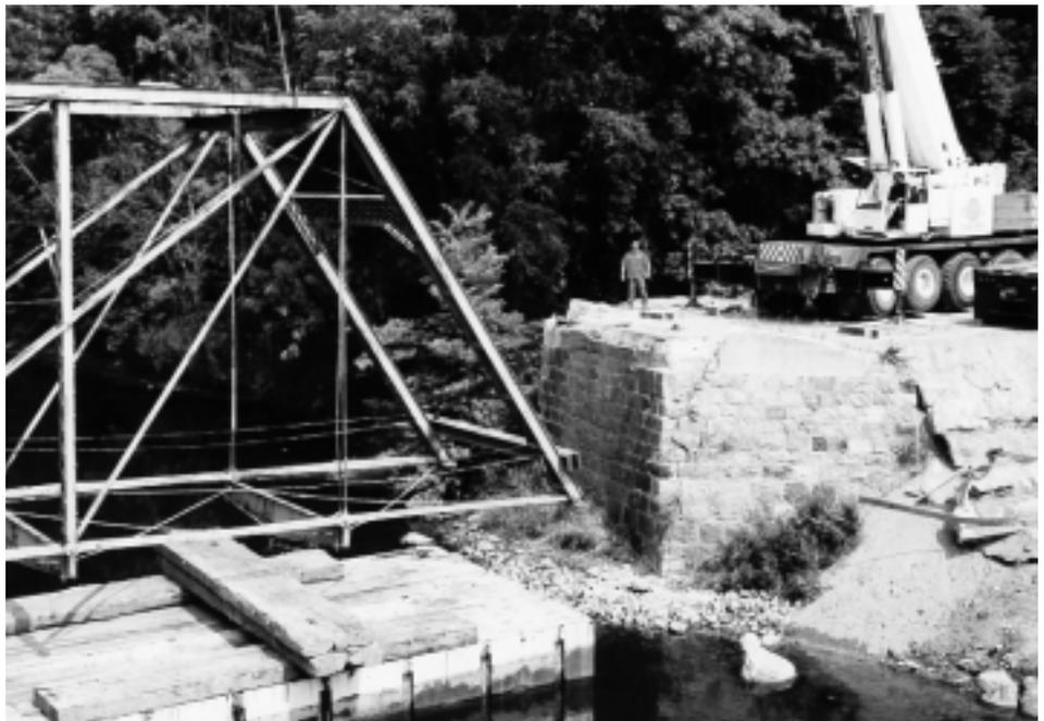
Figure 3. Lifting the Charlotte Highway bridge from its original abutment. This end was lowered onto a barge prior to hauling the bridge across the river and up the other bank.
