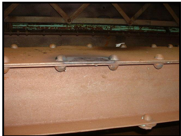
Pack rust removed
