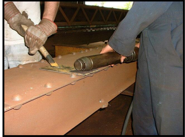
Rivet hammer with modified snap
